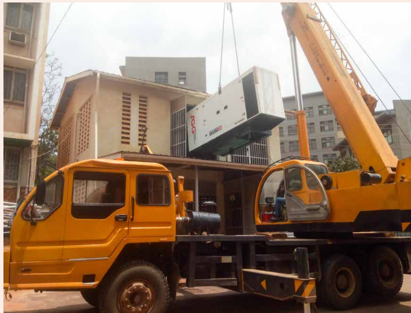
Setting up a Power Generator at the MUWRP Laboratory
