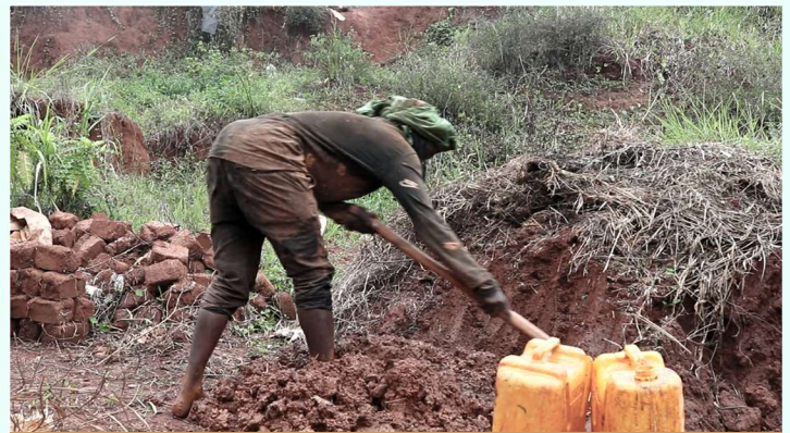
Florence at her brick laying site
